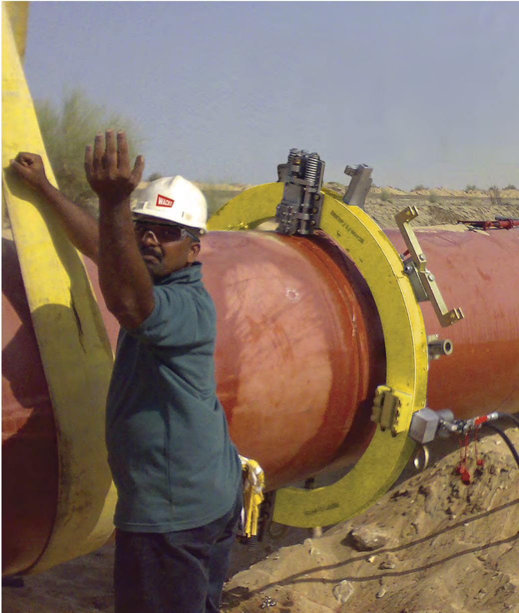
Simultaneously cuts and bevels out-of-round pipe
